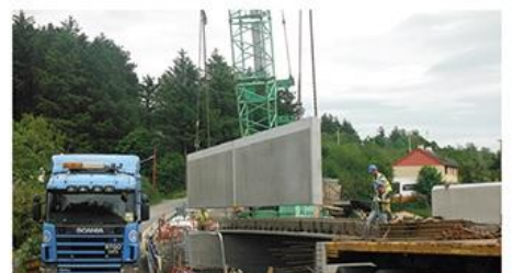
Works at Elactagh Bridge near Cloghan
